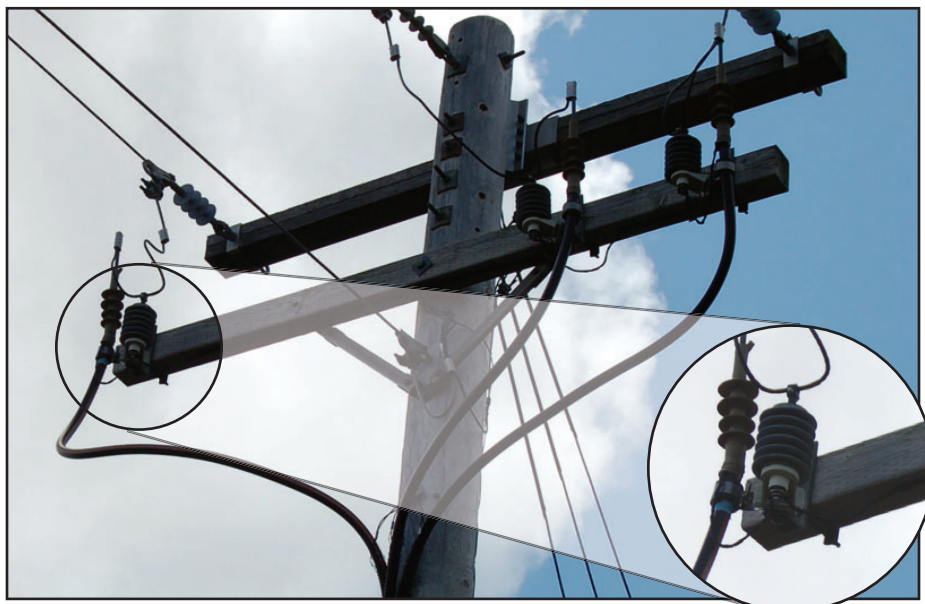
This pole has multiple arresters on it. They divert lightning away from wires leading to an underground service to prevent lightning from causing a cable fault or outage.
