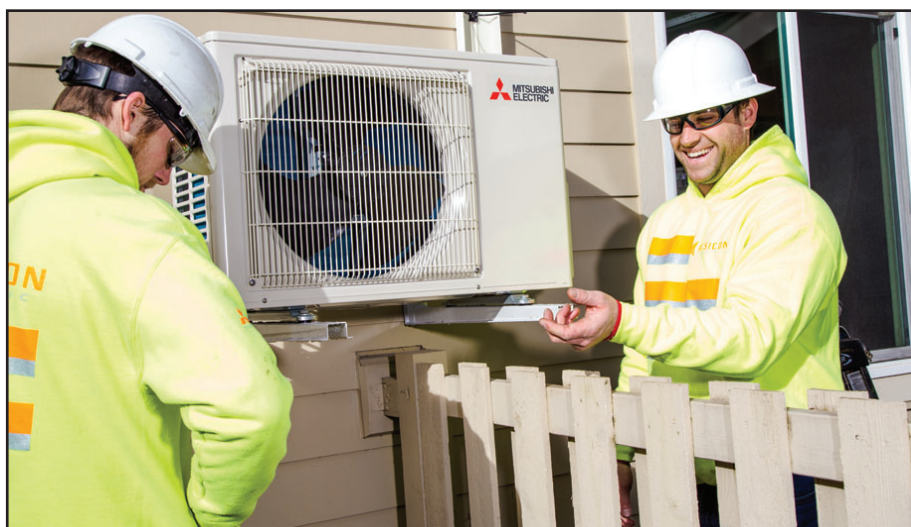
Ductless air-source heat pumps have become more popular in recent years. They are great for homes without ductwork. It consists of an outside unit and an inside unit to reduce your heating and cooling bills dramatically. — Photo by Marcela Gara
