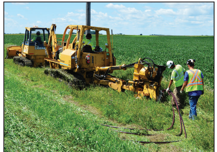
Crew Foreman Mike Suess (far left), Journeymen Linemen Zach Gulden and Brady Kerkhoff and summer helper Kyle Goblirsch (far right) work to upgrade overhead line to underground line in Leavenworth Township. (5)
