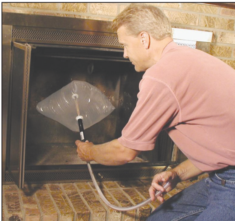
The chimney is a culprit for air leaks if the flue is not working properly. A chimney balloon can seal the opening.
